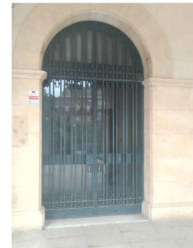
Porta existent tancament E5
